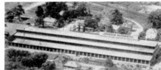
HOME OF JOHNSON AUTOMATICS
